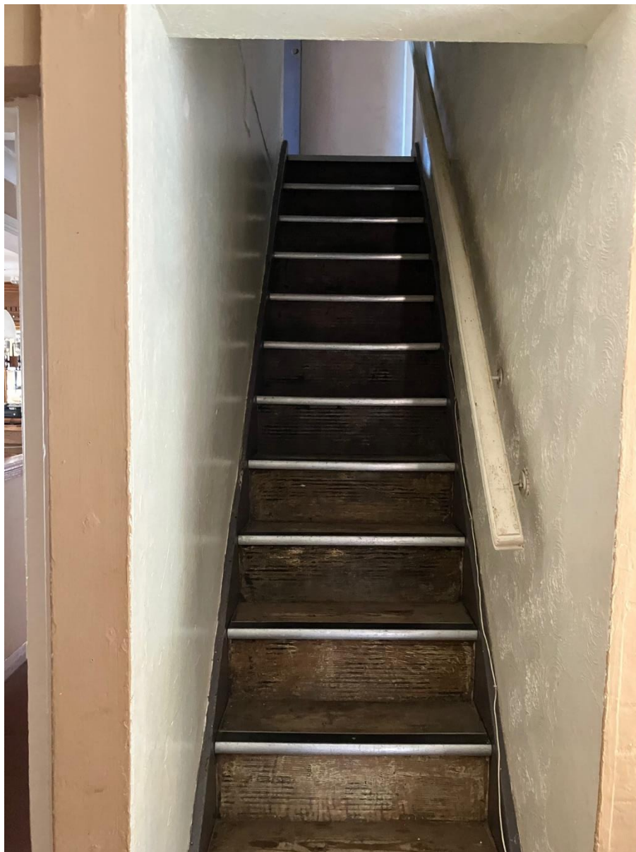
Photo 15 - Steep middle stairs – view from ground floor
