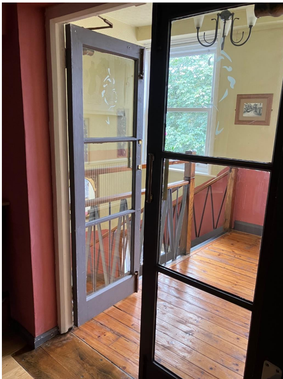
Photo 12 - Doors 1 st floor unused function room looking to front stairs
