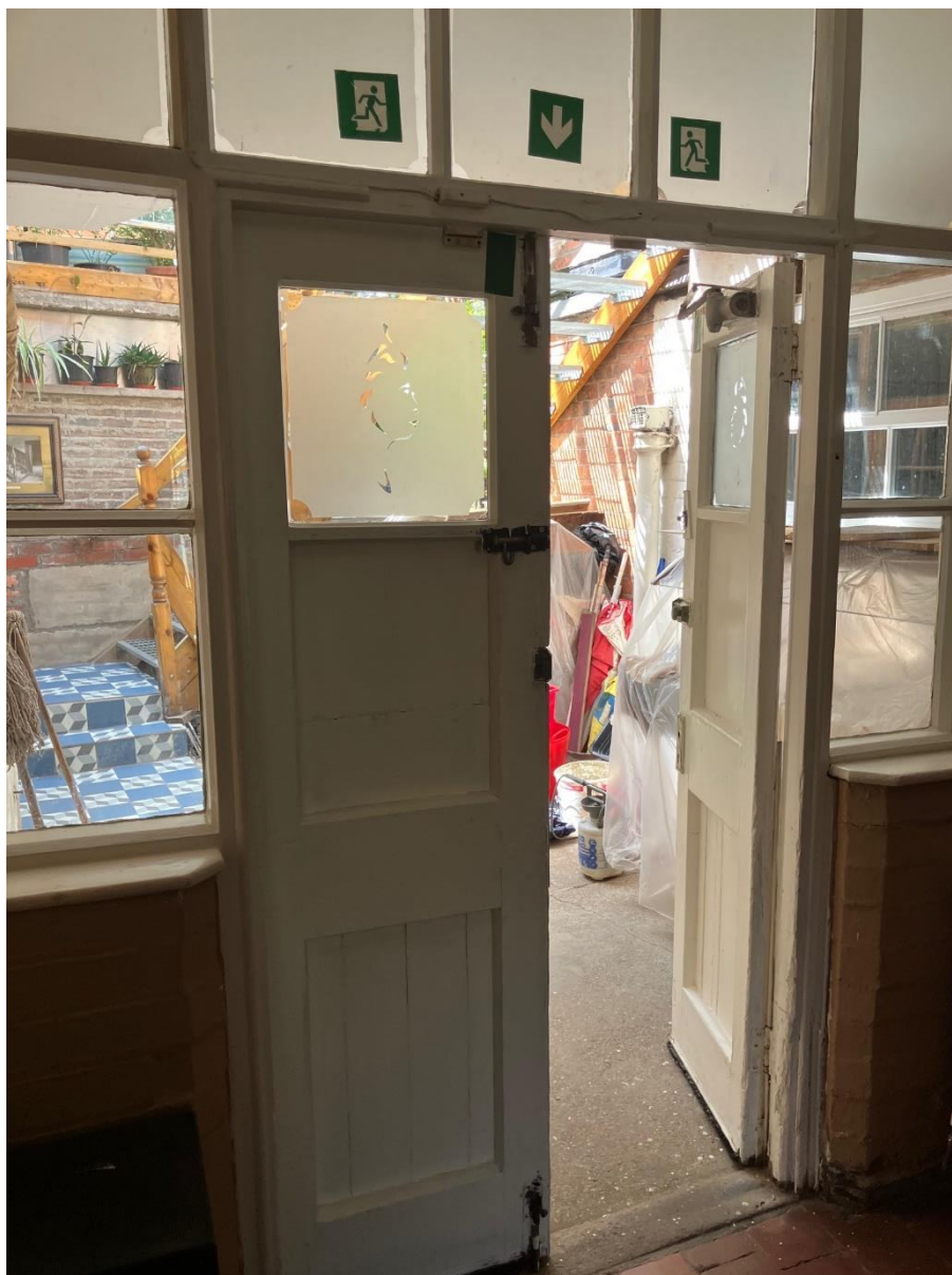
Photo 3 - Fire exit and door leading to rear of premises
