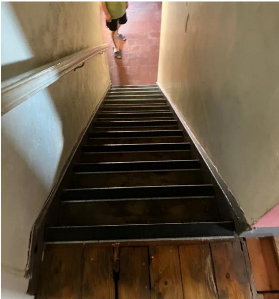
Photo 14 - Steep middle stairs – view from 1 st floor
