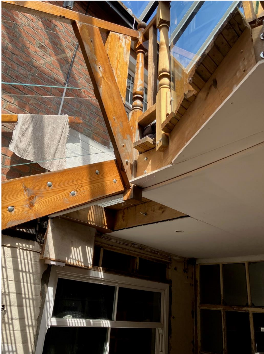
Photo 6 - Balcony area on 1 st floor
