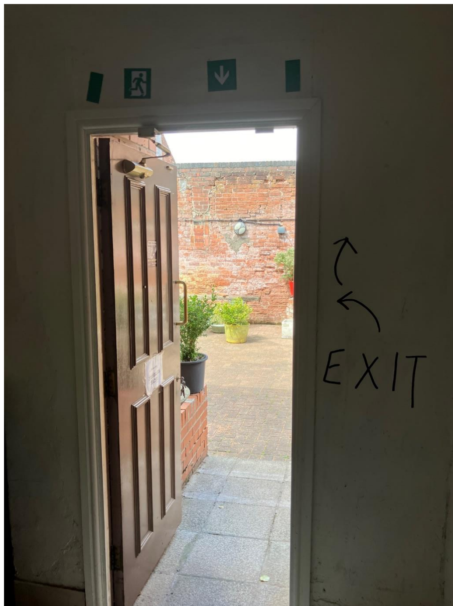
Photo 7 - Side fire exit and door into beer garden
