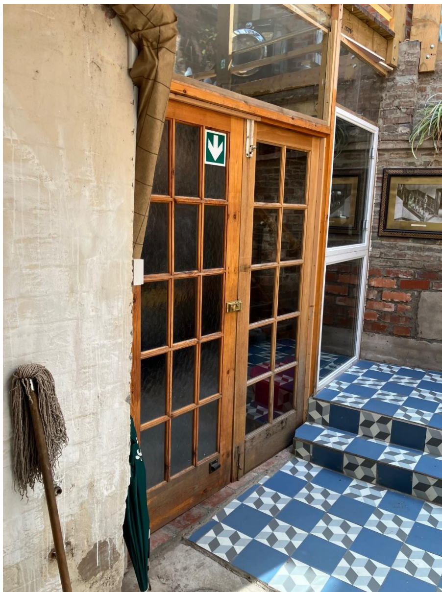
Photo 4 - Covered courtyard area at rear – door and fire exit to carport/tunnel
