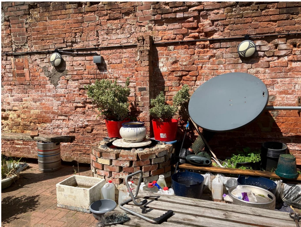
Photo 11 - Lighting and some of the clutter/debris in beer garden
